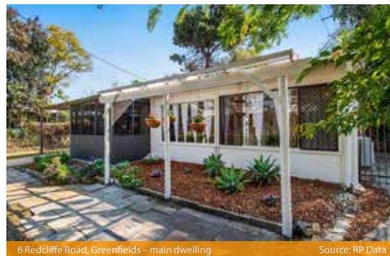
6 Redcliffe Road, Greenfields – main dwelling
